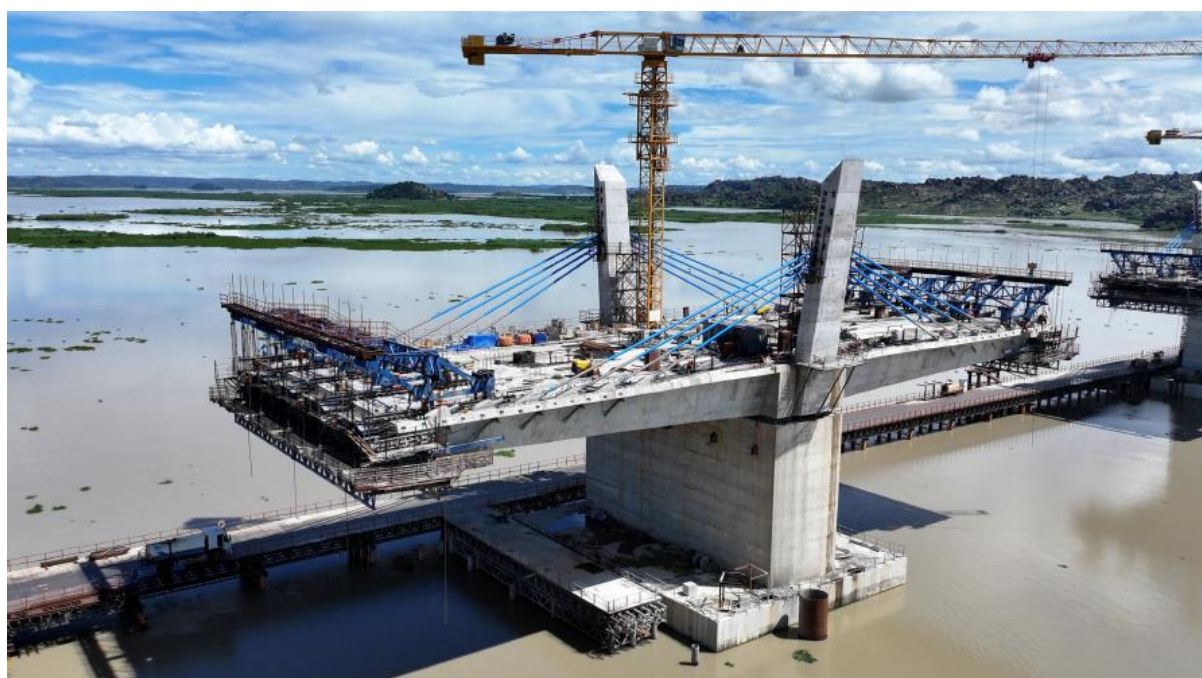
Figure 11: Construction of Pier Table (Zero Segments)
